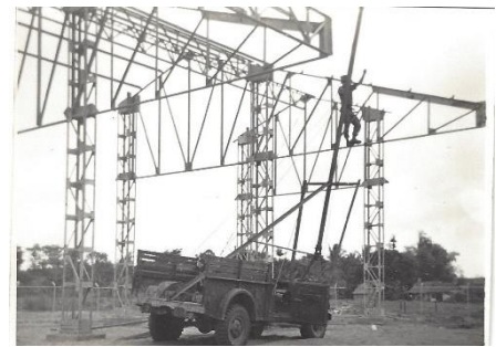
Figure 4- Mobile Crane erecting truss components
