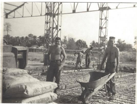
Figure 5-HM2 Miller and CE2 Franks working concrete floor slab
