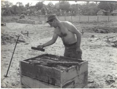
Figure 3 BU2 Karlson placing concrete footing
